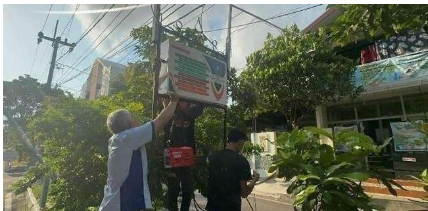
Gambar 1. Proses Instalasi Neon Box
